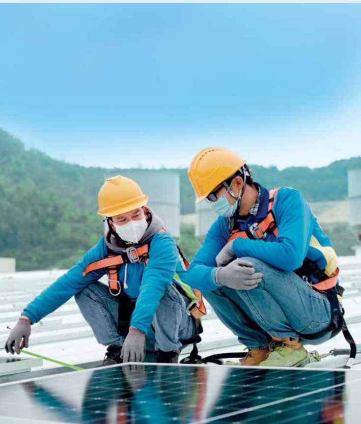
Solar panel installation at Wellcome Fresh Food Centre, Hong Kong
