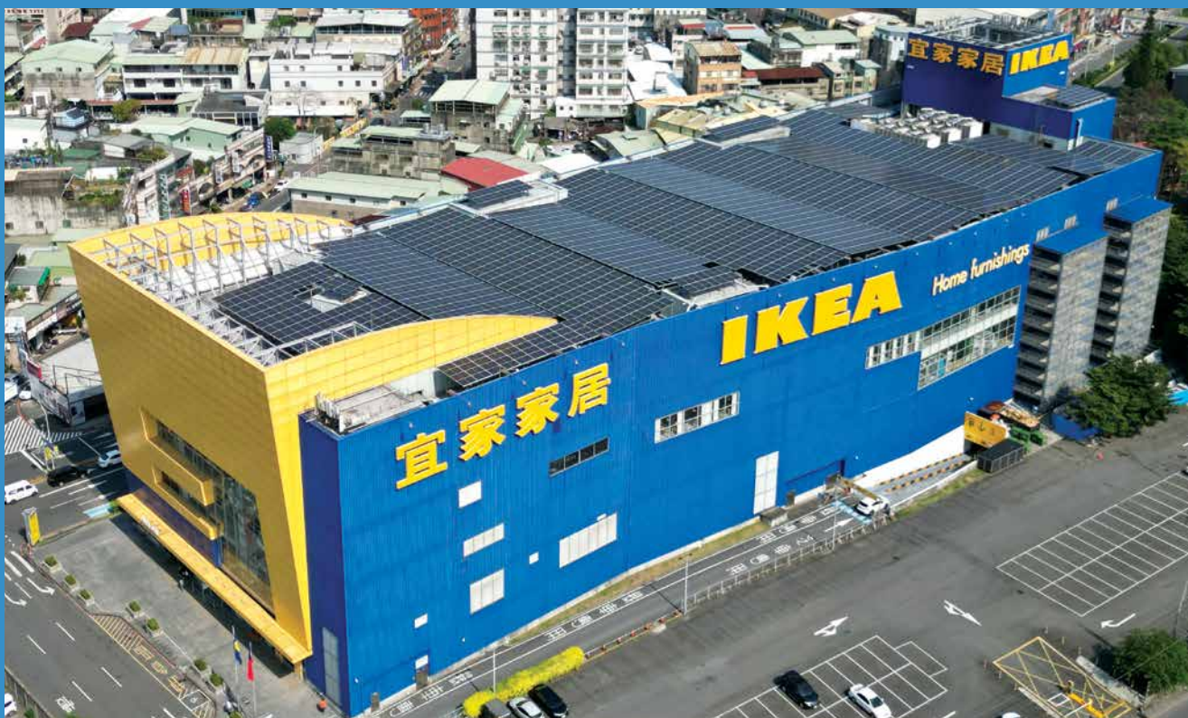
Solar panels at IKEA Hsin Chuang store, Taiwan
